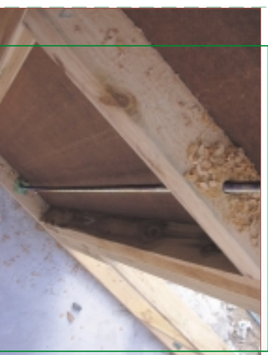
M4 Short Wall requires the addition of M12 anchor rods to achieve its design strength.
