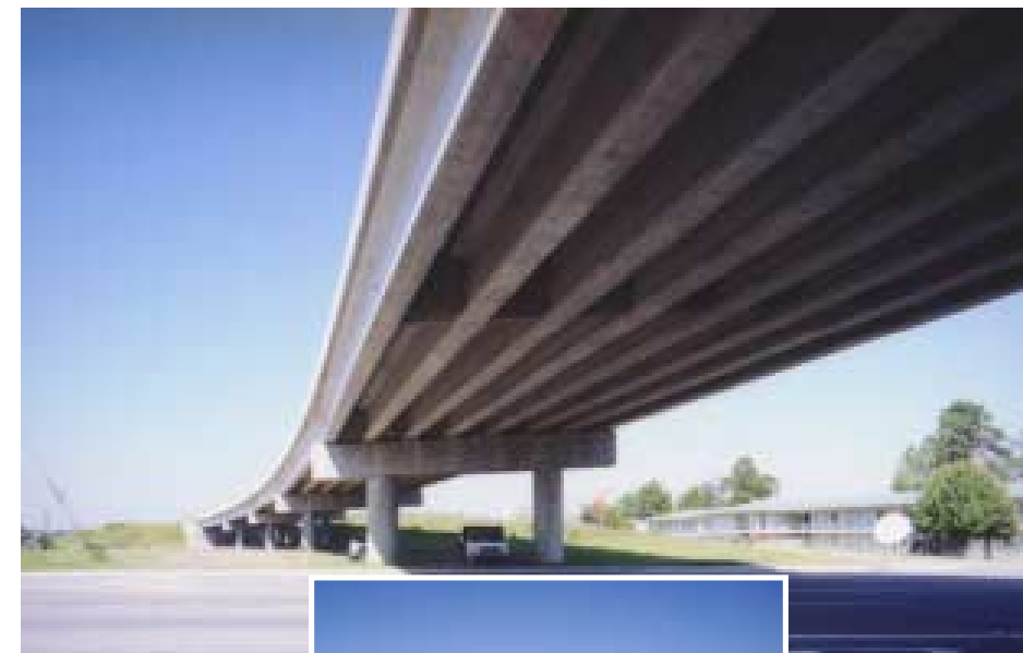
Mark Clark Expressway Charleston, SC
