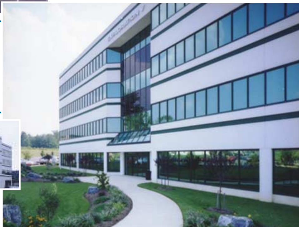
Glenbrook at Westfields and Exploration V utilize Tindall's Total Precast Framing System (beams and columns)
