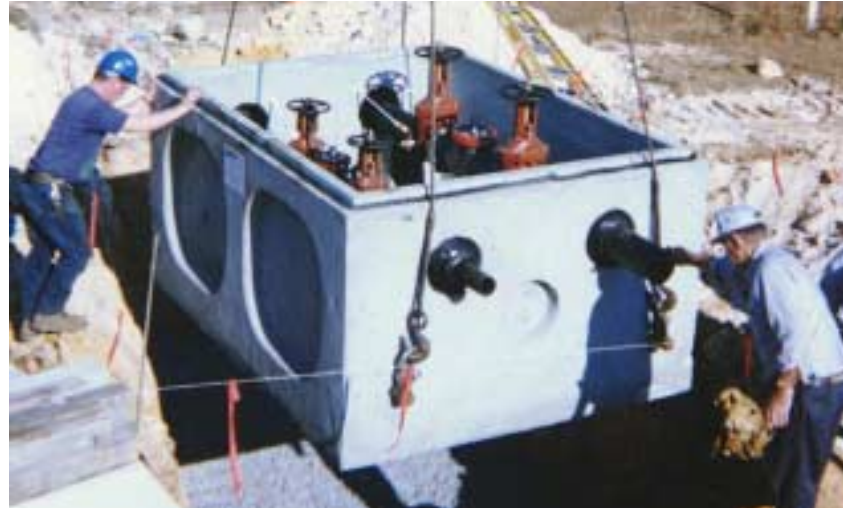
Upfit Valve and Meter Vaults
