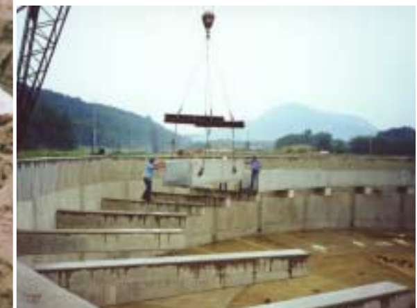
Clarifier Overflow Structures
